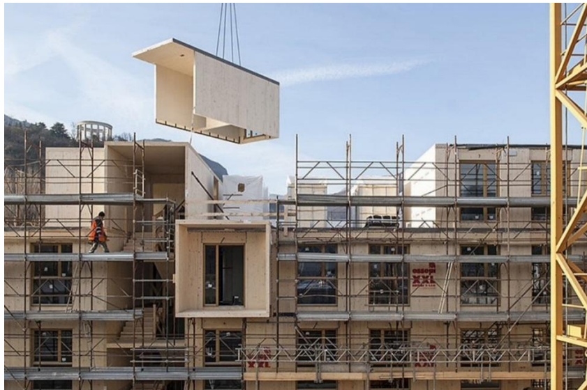
Fig. 2 - Wooden construction sections
