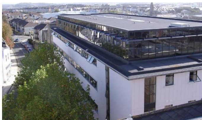
Figure 3 Roof-top extension using modules at Plymouth University, UK
