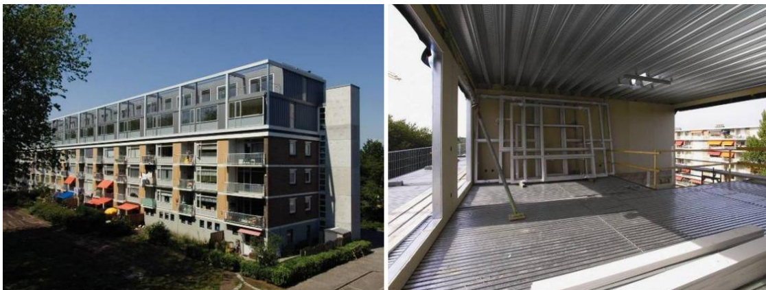
Figure 2 Two storey extension of an existing building using light steel framing
