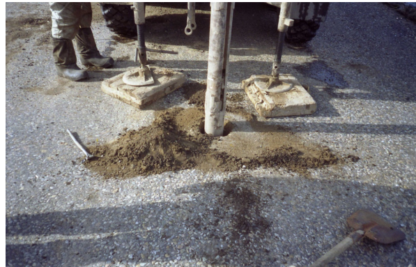
Figure 3 - Machine UGB 50M while drilling with pneumoglass
