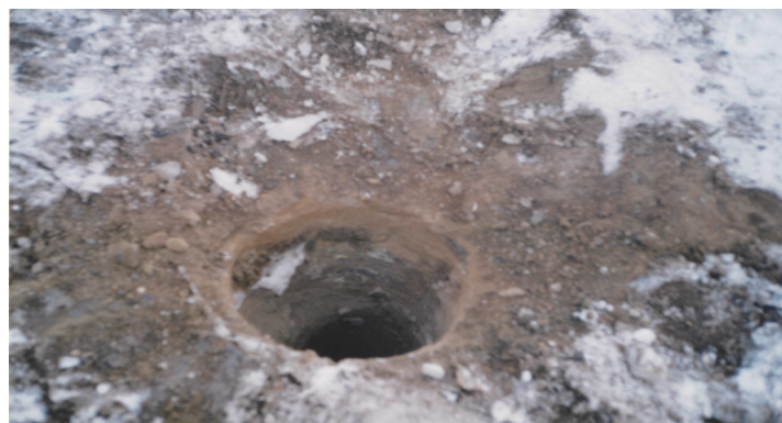
Figure 11 – Drilled road construction till 4 meters depth
