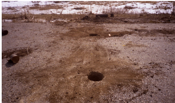
Figure 10 – Drilled road construction in the middle of road and traffic path
